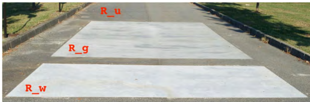
Figure 3. View of the experimental installation, taken in condition of glazing sun lighting quite parallel to the direction of view to emphasize the different behavior of the actual asphalt and coated pavements (from top to bottom: actual asphalt, grey and off-white elastomeric coatings).
